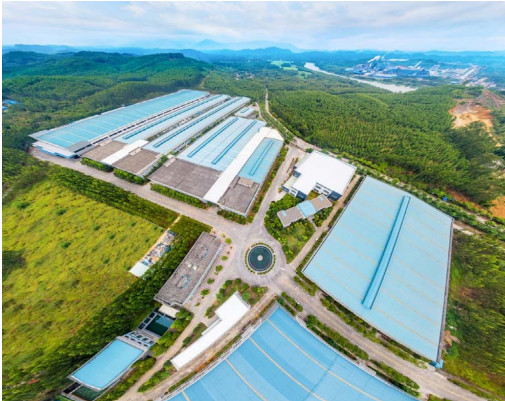
Manufacturing area UAV Aerial Images
